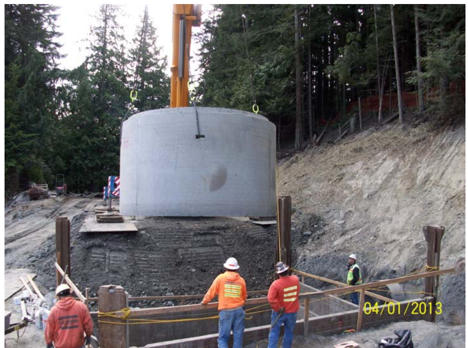
Installing concrete outlet control shaft at City Lake
