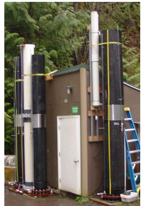
Slow sand pilot filter columns
