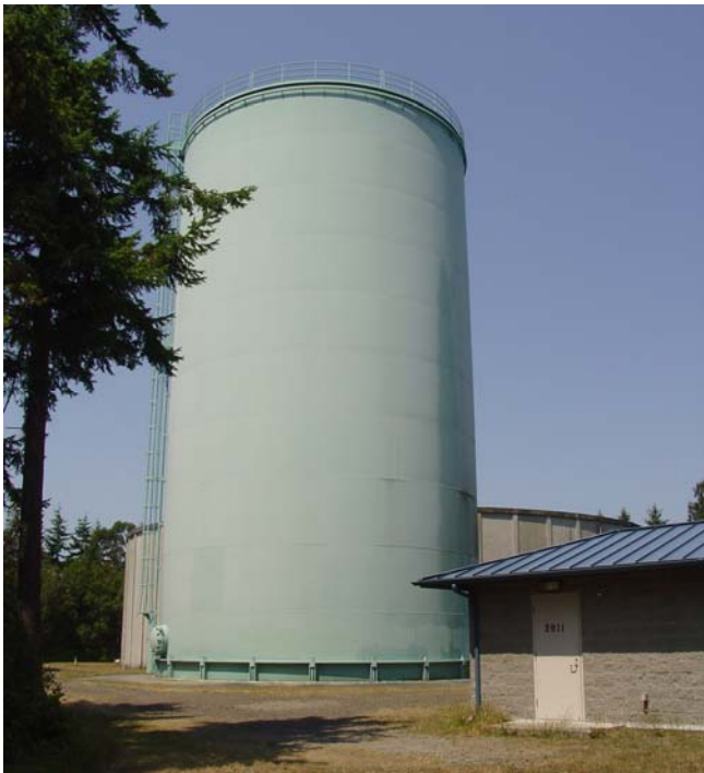
CT compliance station, 1 million gallon standpipe, and 5 million gallon reservoir
