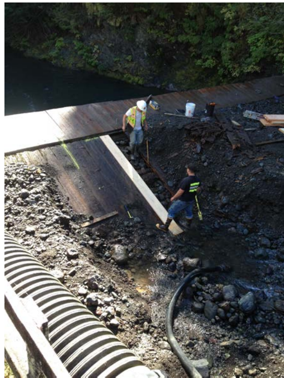
Big Quilcene Diversion Inspection
