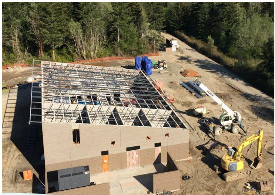
Construction of water treatment facility
