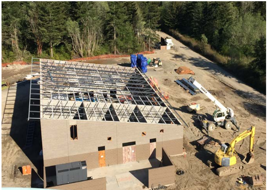
Construction of water treatment facility
